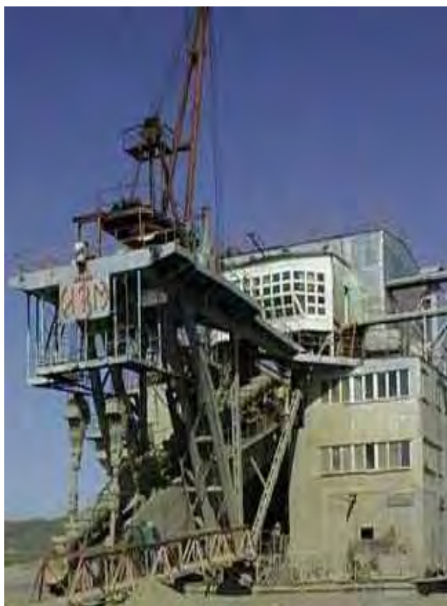
Fig.2: front view of Mongolrosvestmet gold dredge in Zaamar Goldfield in 1998.
