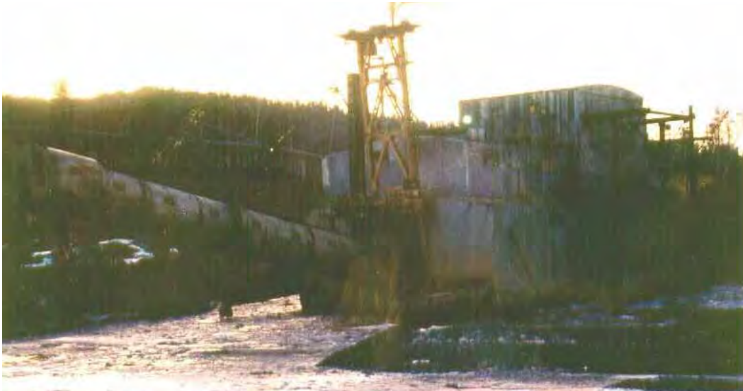
Fig.6: Rear view of Mongolrosvestmet gold dredge in the Yeroo Goldfield in 1998, showing covered boom enclosing conveyor with oversize, and launder chute discharging fines from the sluices. (Photo: Mongolrosvestmet JSC)
