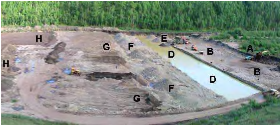
Fig.7: Panoramic view of CGM's Yalbag Mine showing method of mining: A=scrub clearance then topsoil and overburden removed by excavator onto trucks; B=top of placer (pay gravel) cleared of scrub, topsoil and overburden; C=see next illustration; D=flooded excavation of mined-out block, with discharged tailings; E=cones of oversize conveyed into flooded mined-out block; F=cones of oversize burying previous mine-out block; G=trucked overburden being bulldozed over old oversize mounds; H= trucked topsoil being bulldozed over trucked overburden.
