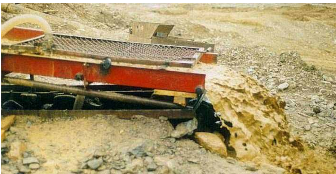
Fig.13: 25m 3 /hour PAuSE NZ Hydraulic Riffled Sluice in action at the Bugant Mine. Note the high clay content of the slurry.
